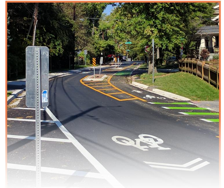
A shared-use lane on one side of Glenbrook Road in Bethesda, with a separated bike lane in the other direction
